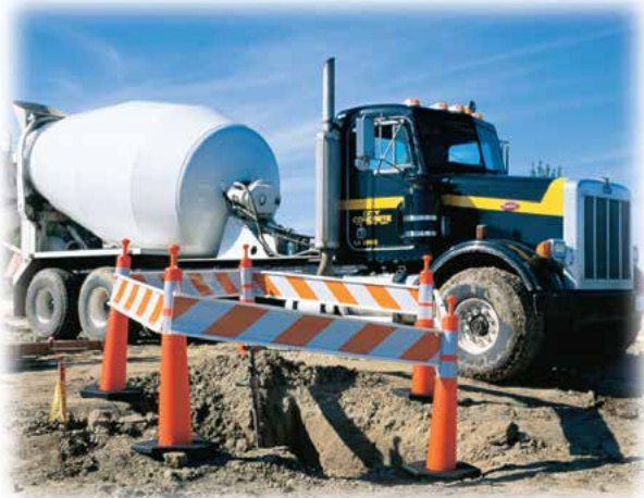
Grabber-Cone 42" and plastic rails can define hazards and construction work areas
